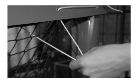
Place the corridors in the middle of the Battery trampolines. Place the frame pads around jumping mats to cover springs. Attach pads to the frame with elastics and belts that are already on the pads and tie them on the frames bellow. Pads that go next to poles have different end that the ones which go around poles. See the photo.
